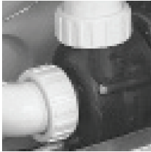
Vent air by slightly opening pump unions.
